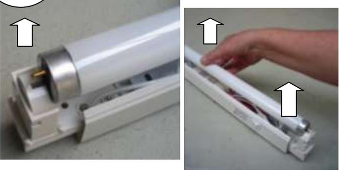
You should now be able to see the pins of the tube are in line with the slot, now pull the tube out holding at both ends
